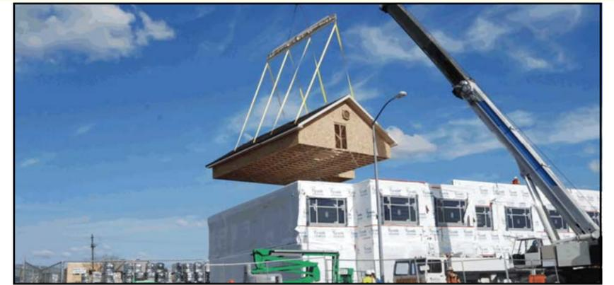
From zero to 21,4480 square feet in less than five days! The new facility at ESD 105 emerged on the south portion of the agency's property during the week of April 12-16. The 22 units of the modular building were constructed in Boise, Idaho, with much of the wiring, plumbing, and other interior features already in place. The new structure is the first modular office facility to be built in Yakima, and will open for operations later this summer.
